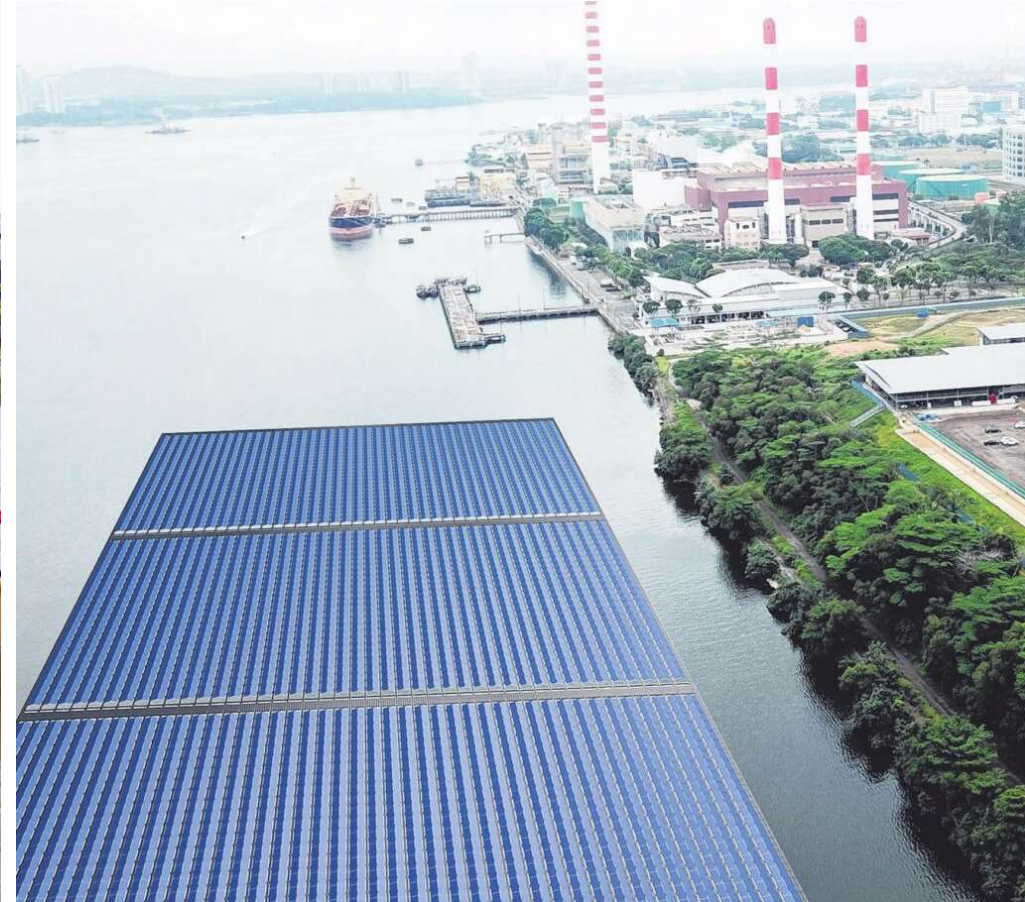
Singapore now home to one of the world's largest floating solar farms. (Source: Straits Times)
